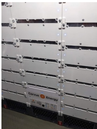
Fig.9. A battery group on board of HaiSea Wamis (Credit: Clear Seas)
