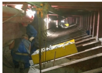
Fig. 16 Pick-hammering the concrete
