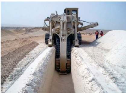
Fig. 2 Equipment-trencher with squeegees
