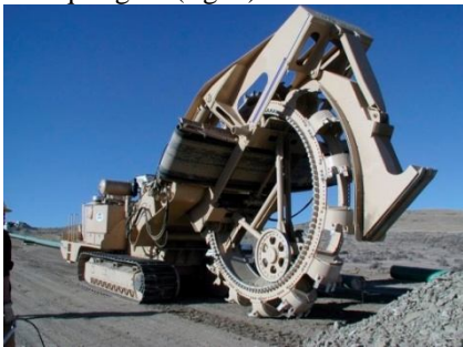
Fig. 1 Equipment-trencher with rotary cup
