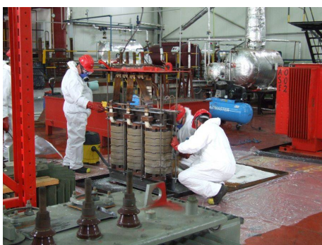
Fig. 2. The dismantling operation of the industrial transformer coil (source: [10])
