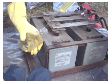
Fig. 3. The method of sampling PCB-contaminated oil from an industrial transformer (source: [12])
