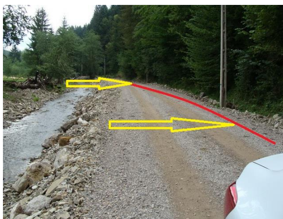
Fig. 5. General view of the Voroneț River shore erosion at the limit of the road DJ 177D in the downstream area after the flood of June 2016 (photo Aug. 2016 [4])
