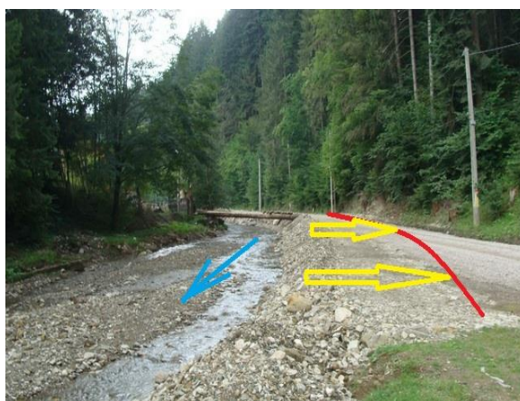
Fig. 6. Details of the Voroneț River's erosive action on the left bank and the road DJ 177D: a - the beginning of the deforestation degradation and the erosion of the road (downstream "Camp Cristea"); b - the end zone of the eroded road section to the slope (upstream of the Brusturosu Brook) [4]
