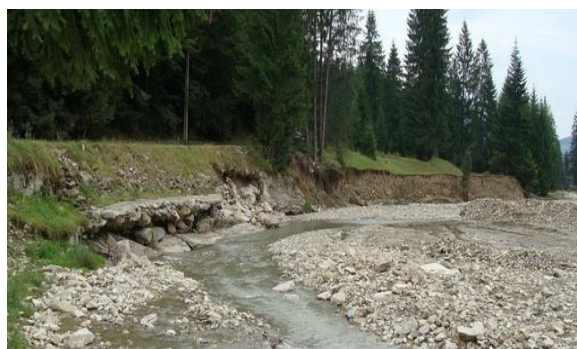
Fig. 5. General view of the Voroneț River shore erosion at the limit of the road DJ 177D in the downstream area after the flood of June 2016 (photo Aug. 2016 [4])
