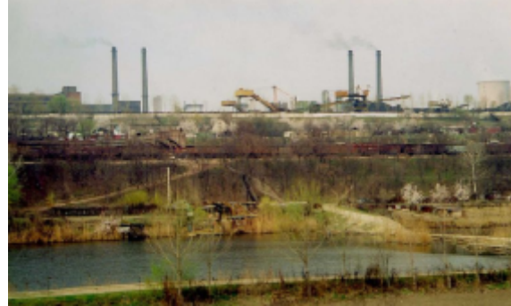
Fig. 3. View of the integrated steel mill plant of Galati (Wikipedia.org)
