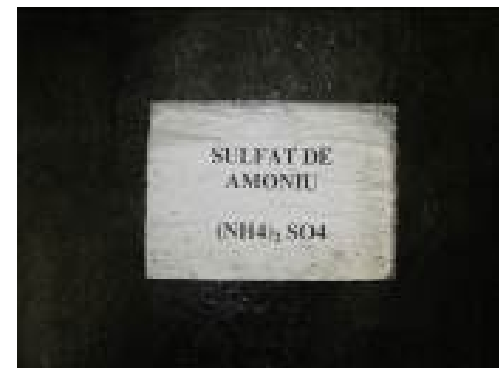
Fig. 6. Tanks with ammonium sulphate resulting from the process
