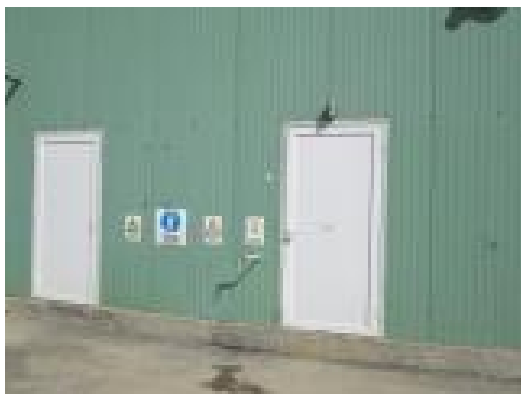
Fig. 2. Room tanks with chemical substances
