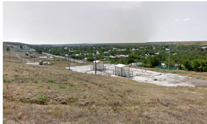
Fig. 5. Illustrative view, at the probes, at the outskirts of the town of Schela, which have sound-absorbing cabs, against the noises
