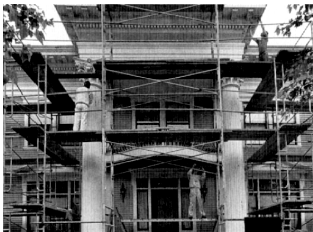
Fig. 4. Process of restoration of facades and column capitols
