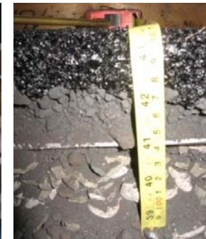
Photo 3, 4. Laying the asphalt coat
