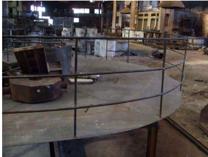
Fig. 3. Image of the casting platform.
