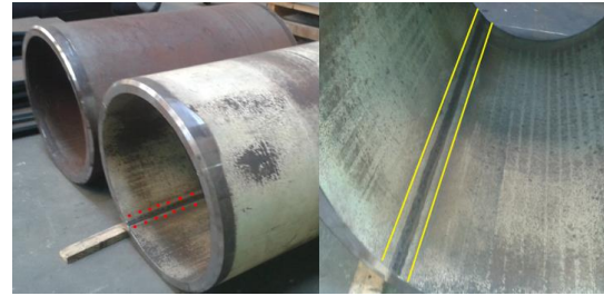
Fig. 16. Completion of the welding operation
