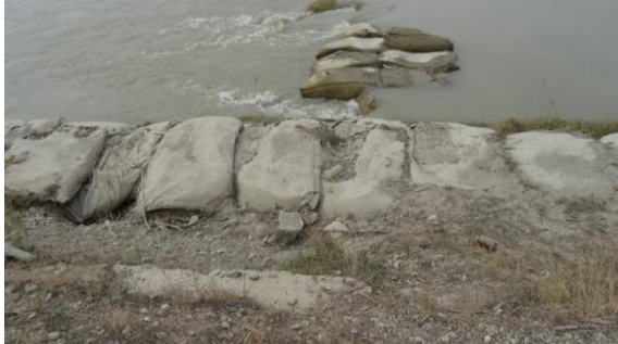
Fig. 15. Details on forms of degradation of geobags under natural and anthropic actions (photo, Sion, 2019)
