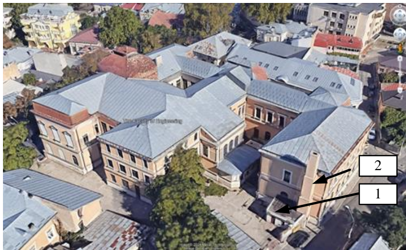
Fig. 1. The headquarters of the Faculty of Engineering and Agronomy in Braila: 1. Heating Plant Room; 2. Flue Gas Stack
