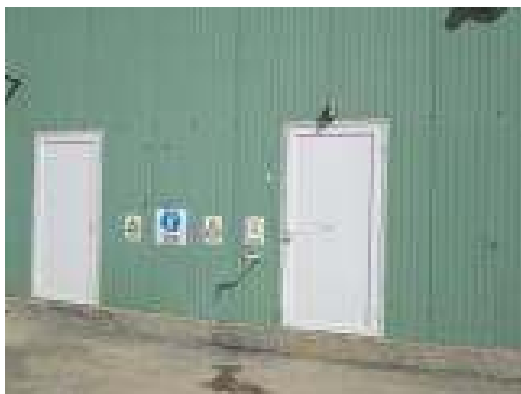
Fig. 2. Room tanks with chemical substances
