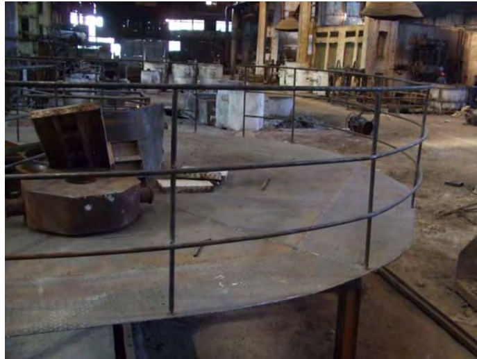
Fig. 3. Image of the casting platform.
