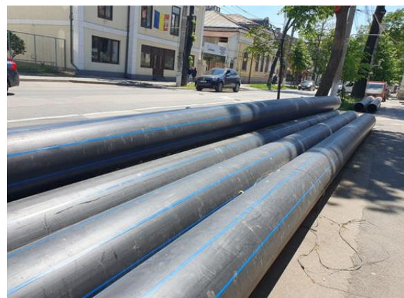
Fig. 5. Polypropylene pipes for the water network
