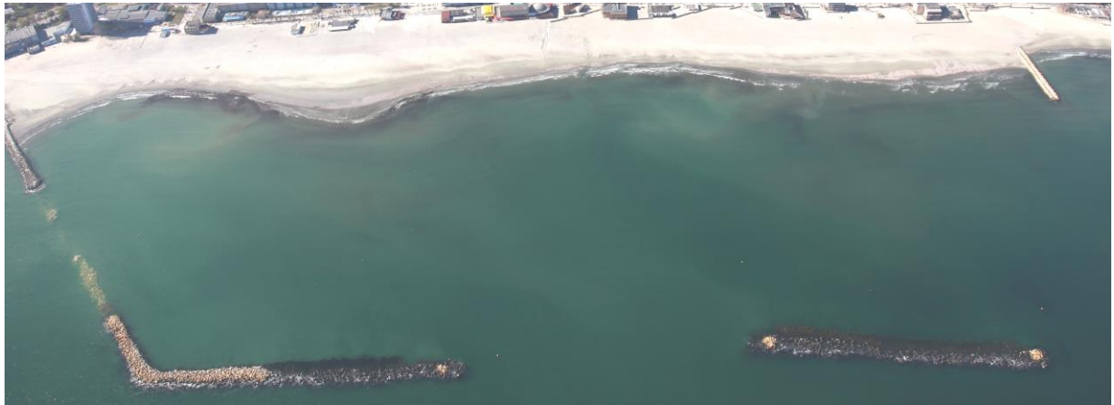
Fig. 4. Dike reconstruction and beach nourishment in the south of Mamaia resort
