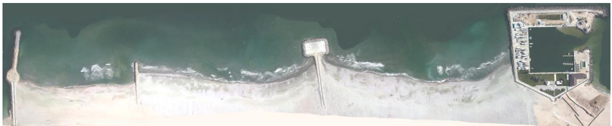
Fig. 5. Dike reconstruction and enlargement alongside with beach nourishment in Eforie North
