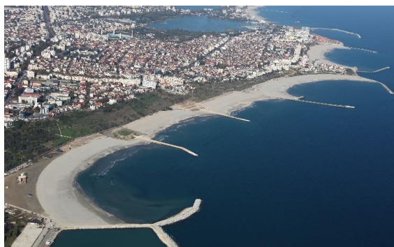
Fig. 5. New dike system constructed and beach nourishment at Constanta
